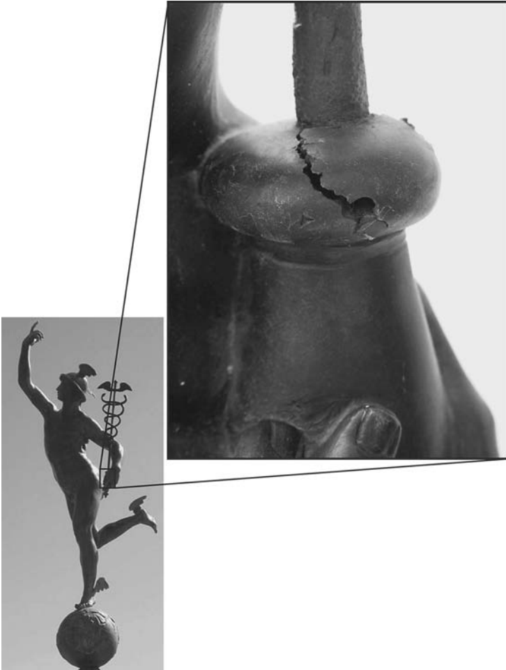
FIGURE 6.46 Stress corrosion crack in a bronze monument caused by buildup of rust around an iron rod. (Courtesy of Kingston Technical Software)
