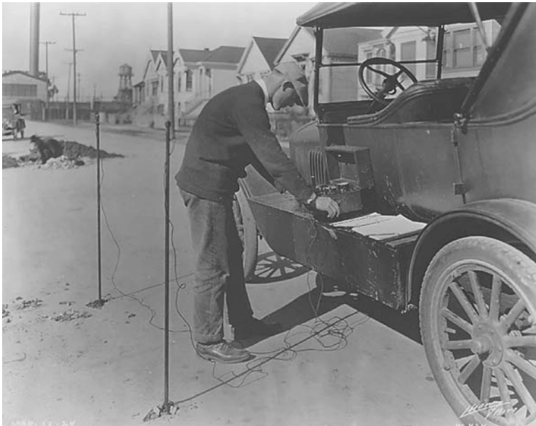
FIGURE 7.4 An electrolysis surveyor using a McCollum earth current meter from the early 1920s. (Courtesy of East Bay Municipal Utility District).
