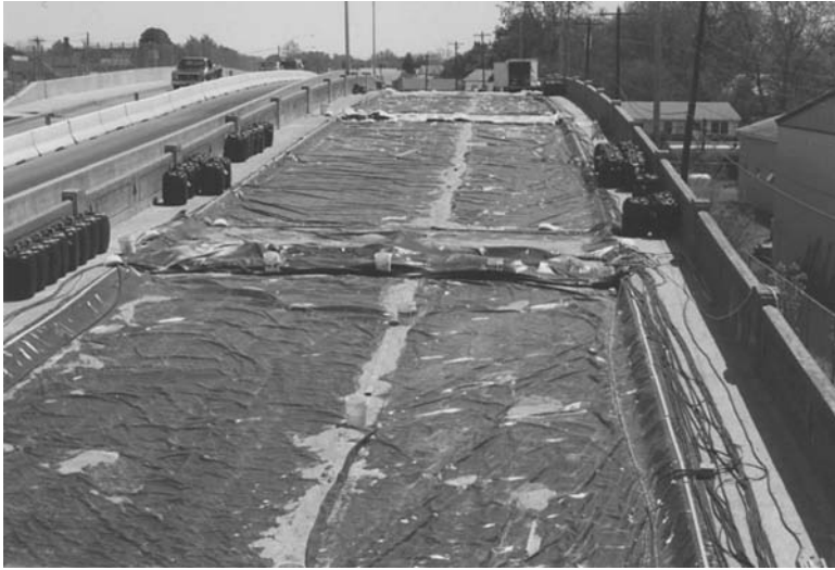
FIGURE 5.46 Bridge deck energized for electrochemical chloride extraction. (Courtesy of Vector Corrosion Technologies)
