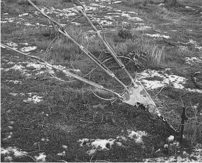
FIGURE 7.14 Typical anchor support with a copper rod ground connection. (Courtesy of Anchor Guard)
